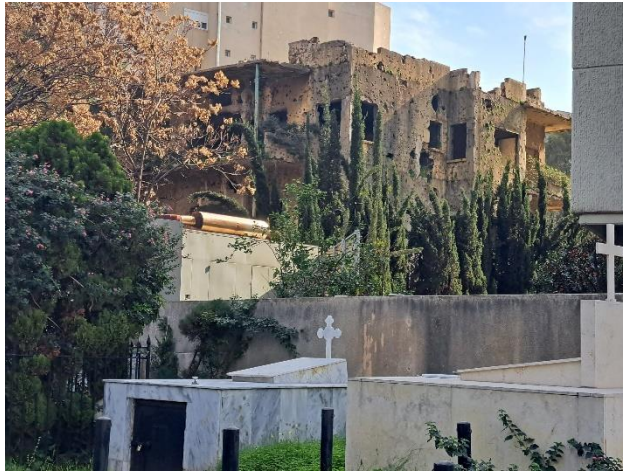
Figure 4. War-damaged building on Beirut's previous demarcation line – Photo Credit: Author N. Hindi – Jan. 2023.
