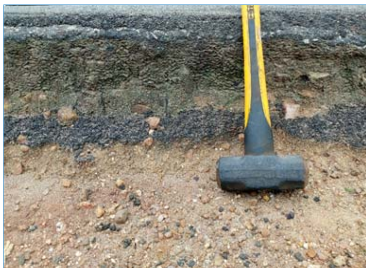
Fig. 10. Section of the exposed highway structure at Ogbese, where existing design thickness was measured to be 315 mm
