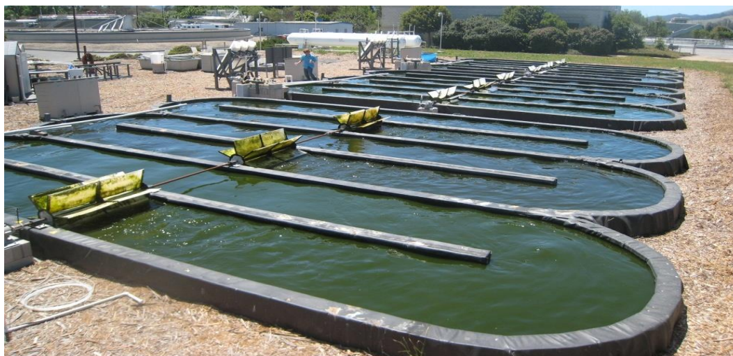
Fig. 7. Use of Algae pounds for water purification.
