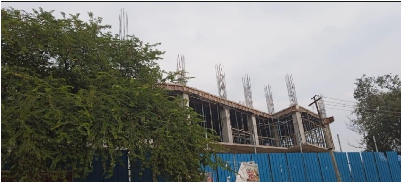
Fig. 16: Recent renovation-construction at the site.
