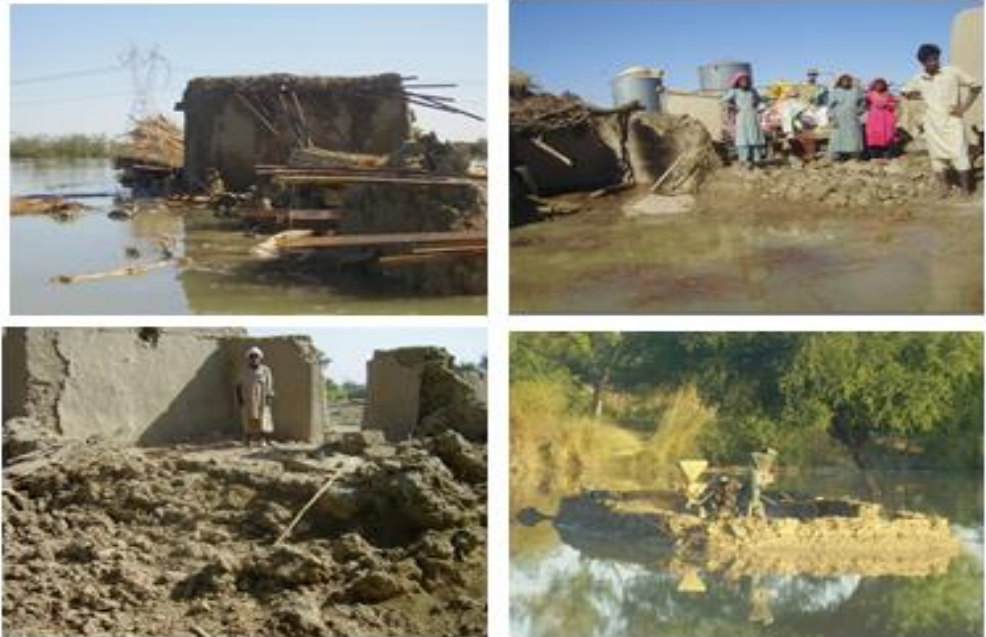
Figure 2. Clay house and prominent damage (Source: RCDS)
