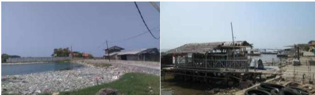
Figure 4. Degradation on the Coastal Edge of Tanjung Pasir Source: Field Documentation (2019)
