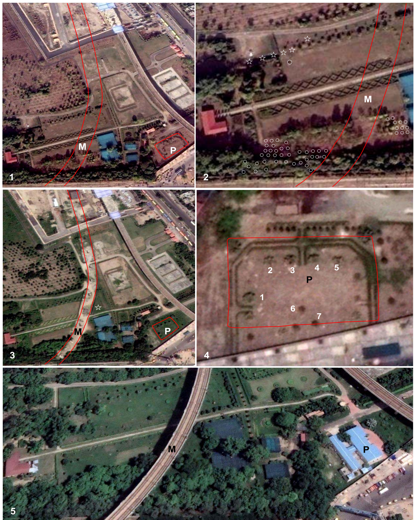
Photo Plate I: 1. Proposed magenta metro lines originating from Botanic Garden Metro Station (M) and construction site of Porta-Cabin for Office-Cum-Interpretation Centre (P), 2. Location of trees/plants transplanted (circle is showing location of transplanted trees from alignment of metro line and star is of transplanted trees from proposed area of Porta-Cabin), 3. Foundation of 9 piers developed within the alignment for metro route, 4. Root balls of 7 trees at site of Porta-Cabin were made for transplantation, 5. Evident luxuriant growth of transplanted trees even after 5 to 7 years and developed metro line (M) and Porta-Cabin (P).
