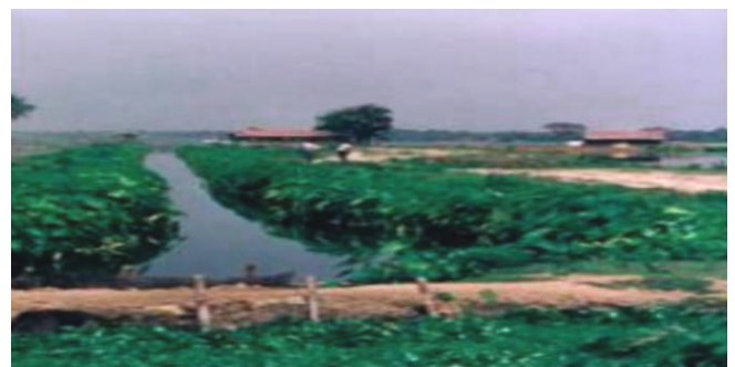
Fig 6: Open channel through which sewage is flown into pond
