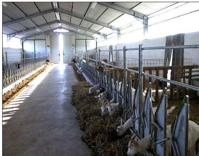
Fig. 3b: Goat concrete house (inner view).
