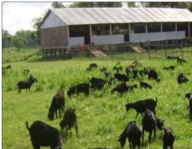
Fig. 3a: Goat concrete house (outer view).
