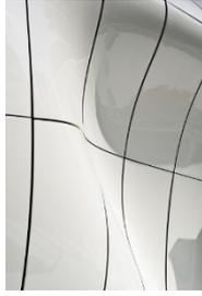
Gambar 34. Kaca Fibre Reinforced Concrete (GFRC)
