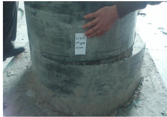
Figure 1: Removal of CFRP wrap horizontally from north face
