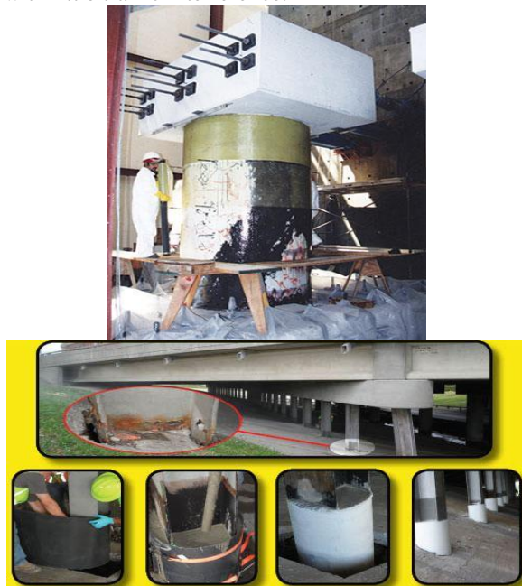
Figure 2: Seismic retrofitting of a bridge with FRP composites.
