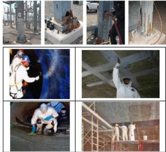
Figure 1: Repair and strengthening.
