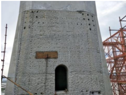
Figure 3.1.1. Construction surface chipping effect diagram
