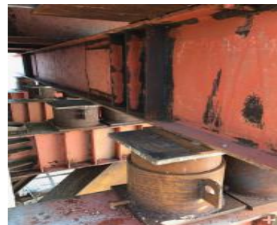
Figure 3.2.2. Setting of support sandbox
