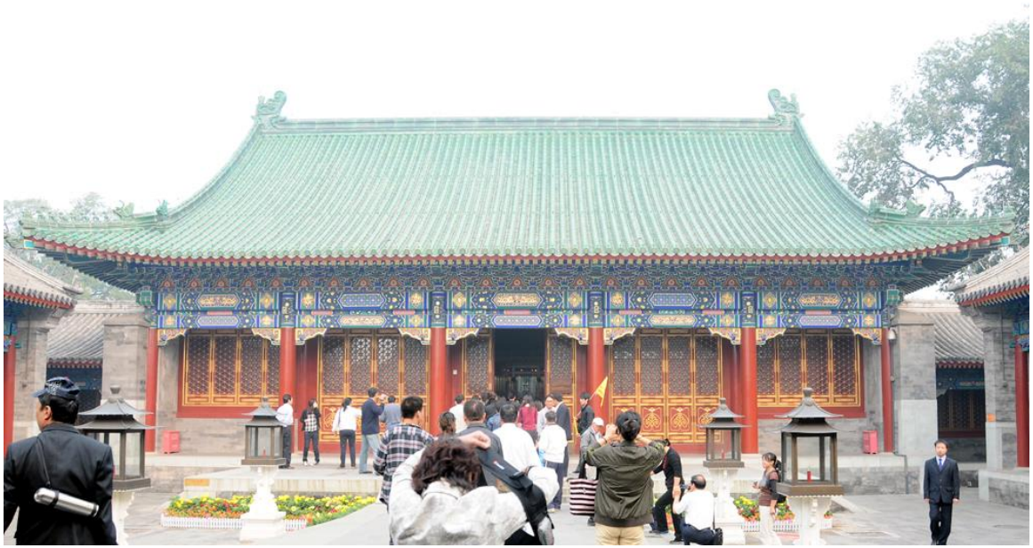
Figure 14. Yinandian at Prince Gong's Mansion ( Gong Wang Fu ) in Beijing has green glazed tile roofs. Photo by Junmin Zhang 2010, print with permission
