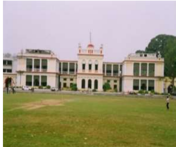
Figure 11 Dutch Structure in Patna
