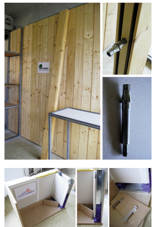
Fig. 4-7 - Geberit System for the assembly of removable toilet cisterns, adapted to create disassemblable internal partitions with metal frame and wooden panels; Gyproc System for disassemblable internal partitions in wood and plasterboard with modular interlocking elements; Systimber System for disassemblable walls in solid tongue and groove wood elements joined with metal connectors; Saint Gobain System for disassemblable internal partitions in plasterboard with dry joints with a cavity behind the baseboard for the passage of the systems. All the Systems have been tested in the Circular Retrofit Lab at the VUB Campus in Brussels (credits: P. Altamura, 2019).
