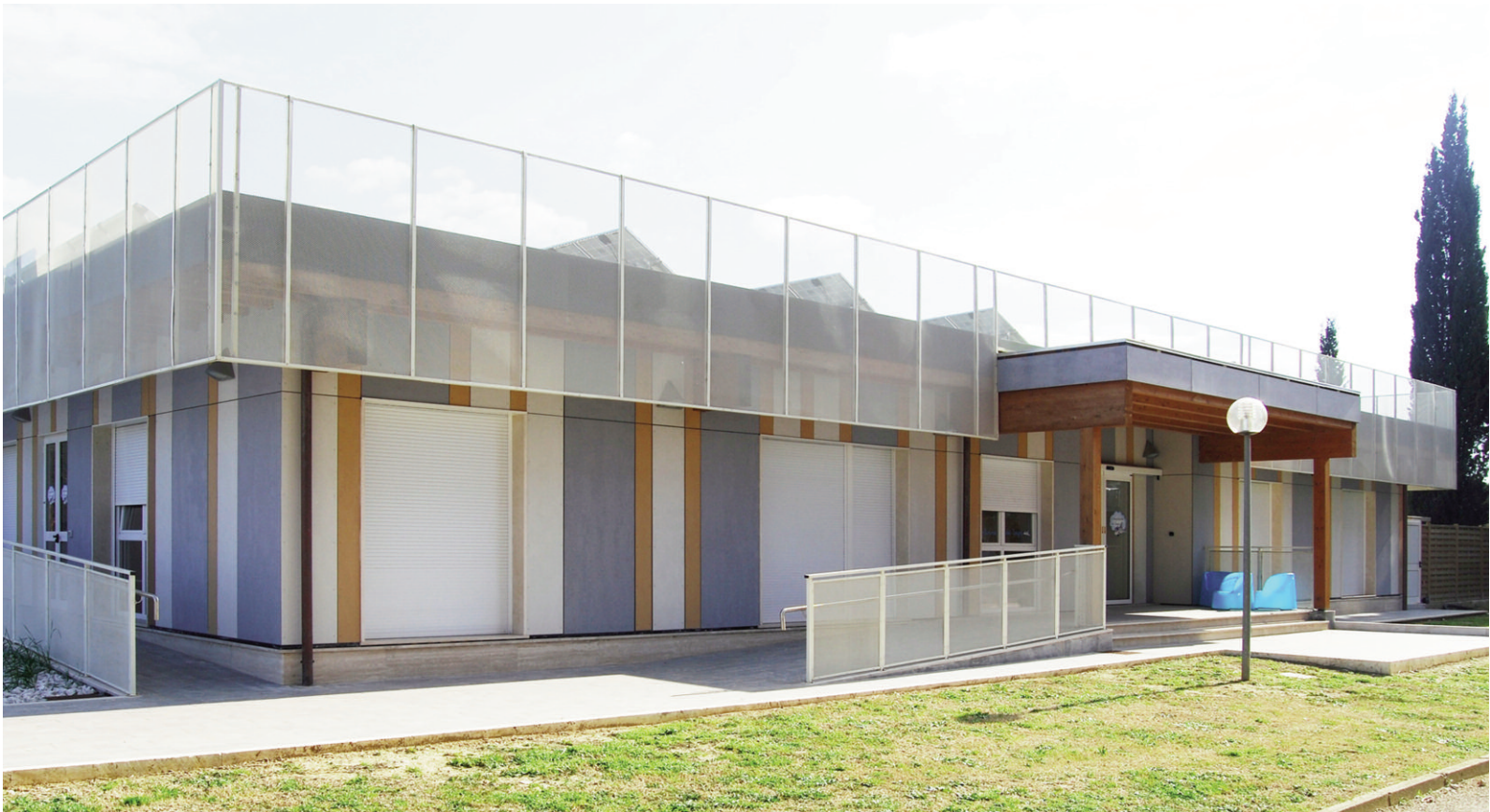
Fig. 8 - Overall view of the kindergarten building built in compliance with the GPP CAM for Buildings at the Grosseto Military Airport (credit: P. Altamura, 2019).
