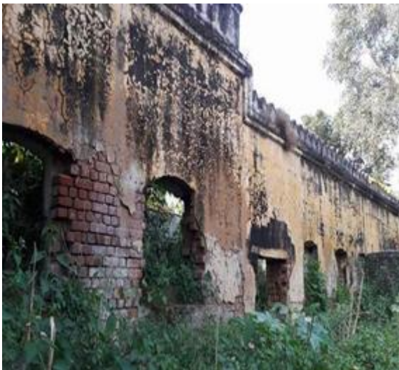
Figure 3 a) Damages to External walls
