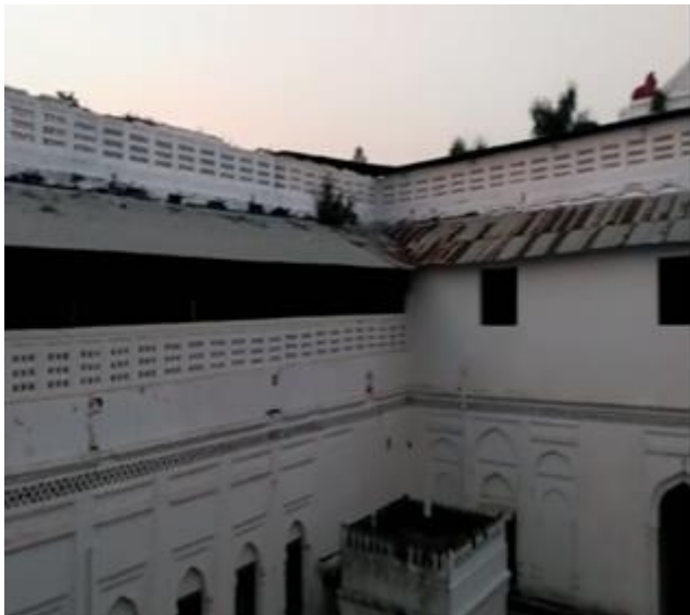
Figure 6 a) Plant growth at the edges of roofs and parapet Figure 6 a) Plants and algae attack
