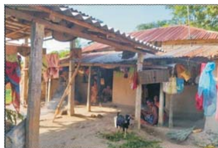
Fig 12: Dilapidated Housing, Humgarh
