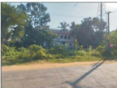
Fig.11: Good Housing Condition, Humgarh
