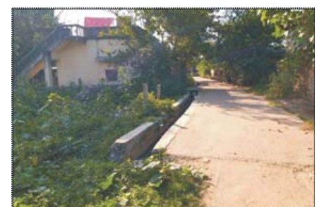
Fig 16: Open Drainage, Humgarh
