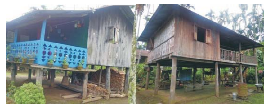
Fig. 5: Timber used as Housing Material (Gangutia Forest Village)
