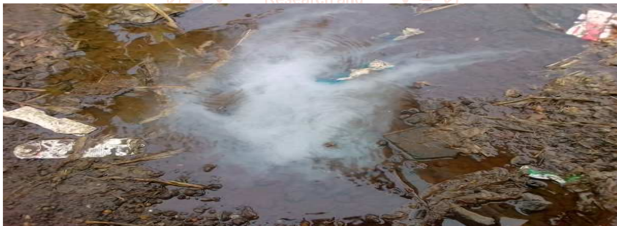
Figure5; A broken and leaking pipe leading to households
