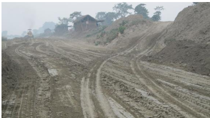
Figure 5.2 Leveling of Road (NH-31)
