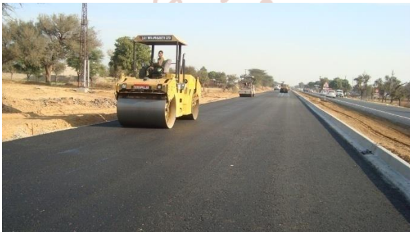
Figure 5.7 Bituminous Macadam (NH-31)
