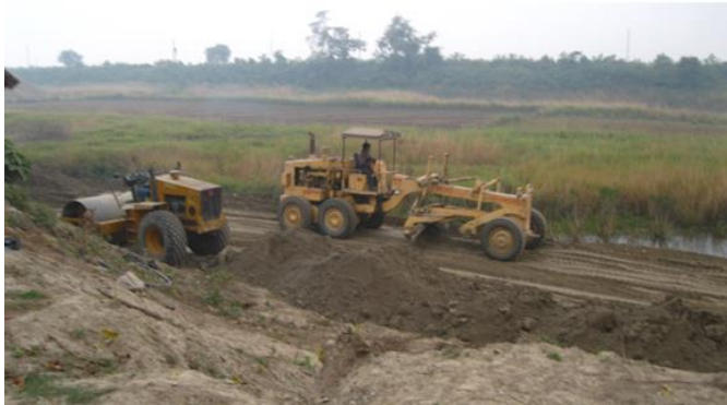
Figure 5.1 Road Excavation (NH-31)
