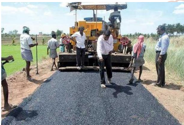
Figure 5.6 Tack Coat (NH-31)
