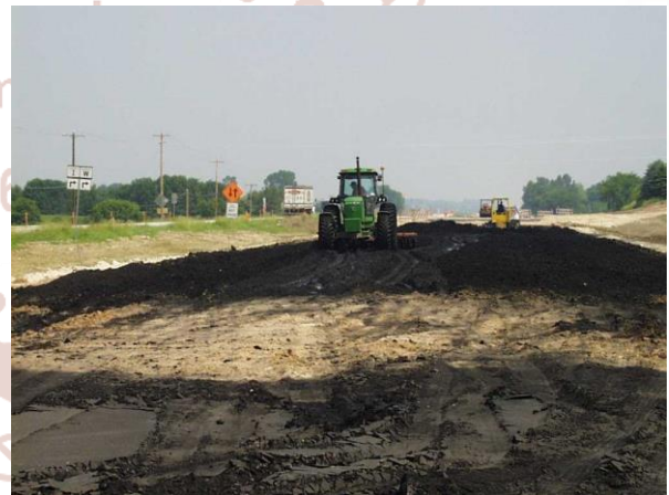
Figure 5.3 Granular Sub-Base (NH-31)
