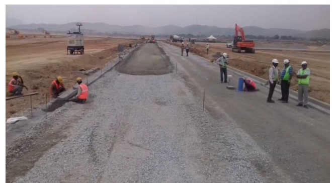
Figure 5.4 Wet mix Macadam Sub-base/Base (NH-31)
