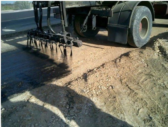
Figure 5.5 Prime Coat over Granular Base (NH-31)
