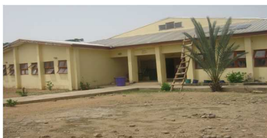
PLATE 3 GOBBIYA PRIMARY HEALTH CARE FACILITY
