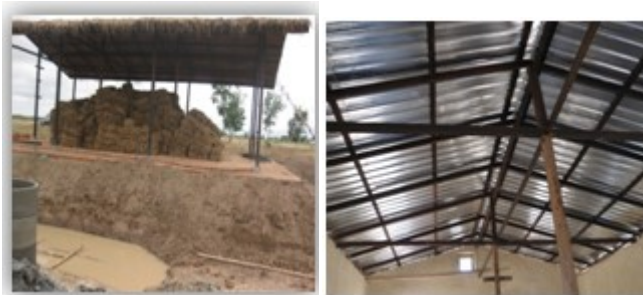
© Fixing of Post and C.G.I Sheet Roofing
