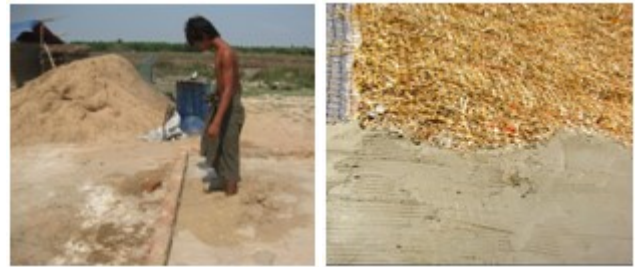
(e)Plastering in (1:3) Lime Mortar
