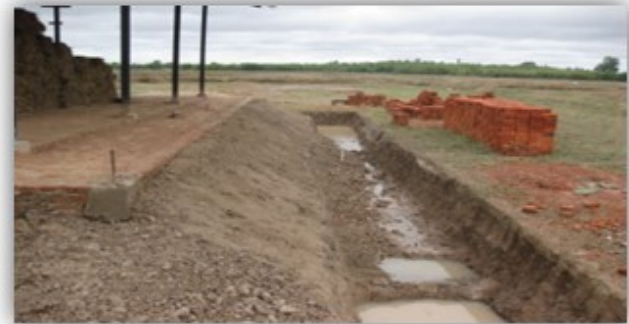
(b) Construction of Foundation
