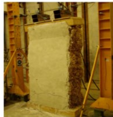
Fig. 9 Lime rendered wall failure
