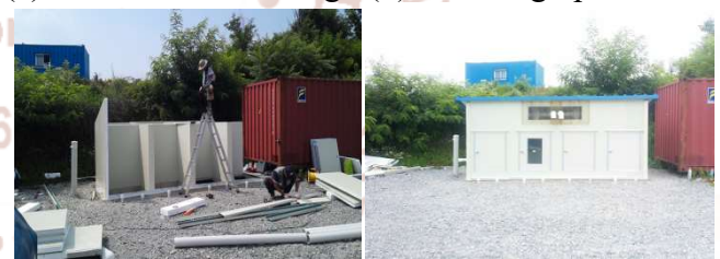
(e) Building of sandwich panel (f) Model house completion
