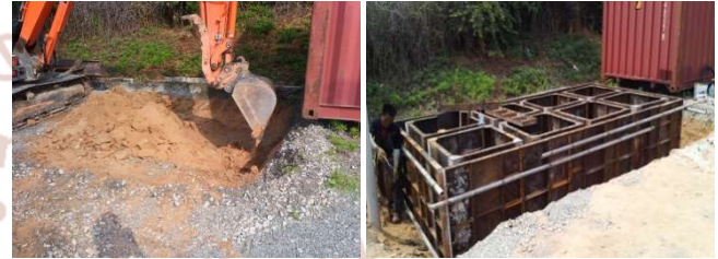
(a) Excavation work (b) Molding
