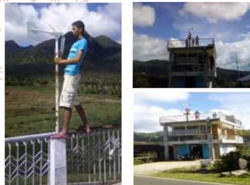
Rooftop installation and testing
