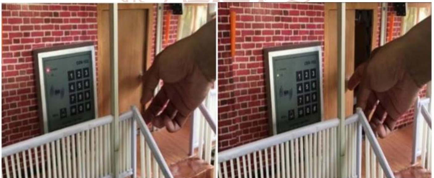
Figure14. Test and Result of Main Door Access Control System
