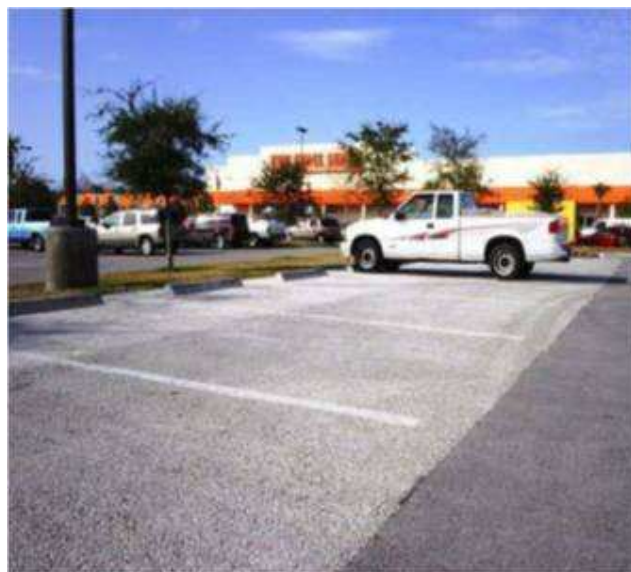
Fig 1.4 Gap graded concrete parking
