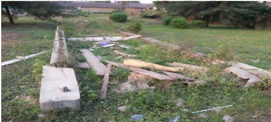
Plate 3: Broken Path Way at Green Grass Park
