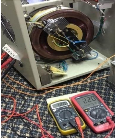
Figure 10. Photo showing 7kVA, Automatic Voltage Stabilizer Control System at under-voltage Condition
