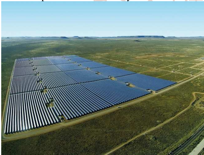
Fig 4 Solar Panel Power Plant
