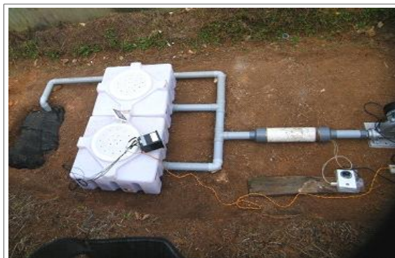
Fig. A : Heating coil arrangement for circulation of hot air during curing
